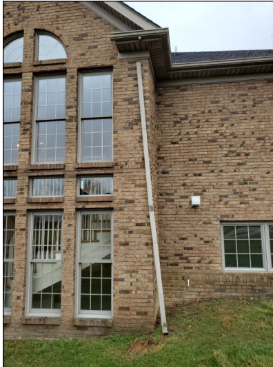
Downspout Disconnected
