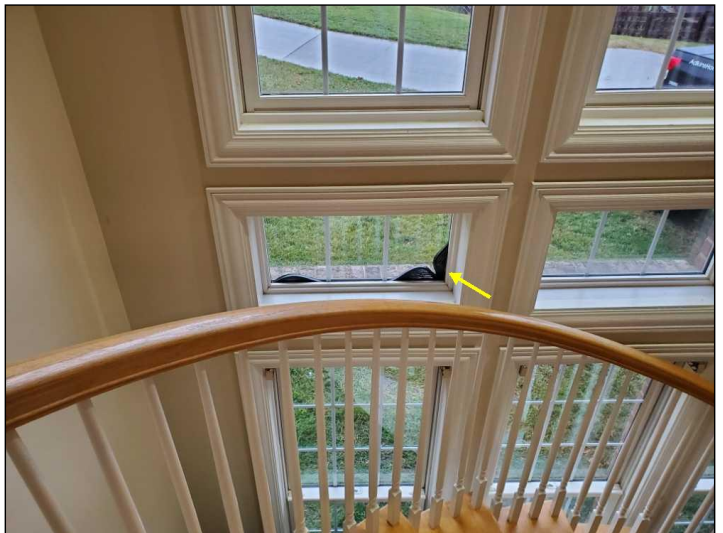
Damaged seal
