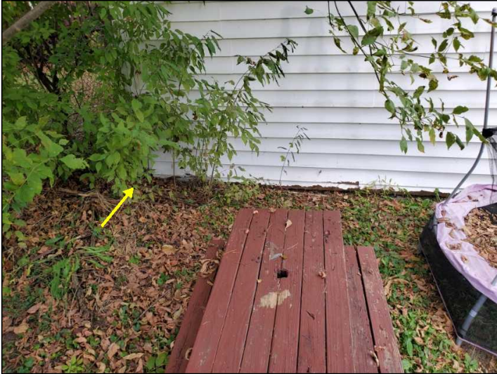
Wall below grade
