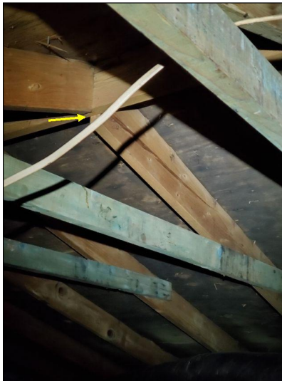
Damaged rafter
