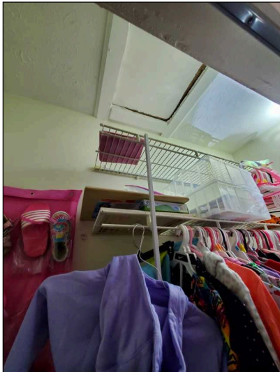
Attic access - Middle bedroom closet
