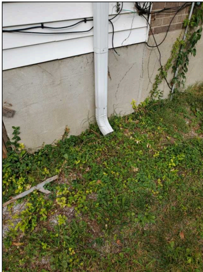
Discharges Near Foundation
