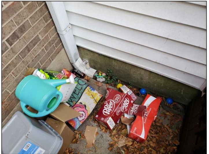
Discharges Near Foundation
