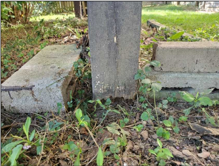
Wood deterioration
